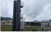
沼气净化加压装置 Biogas purifying compressor
